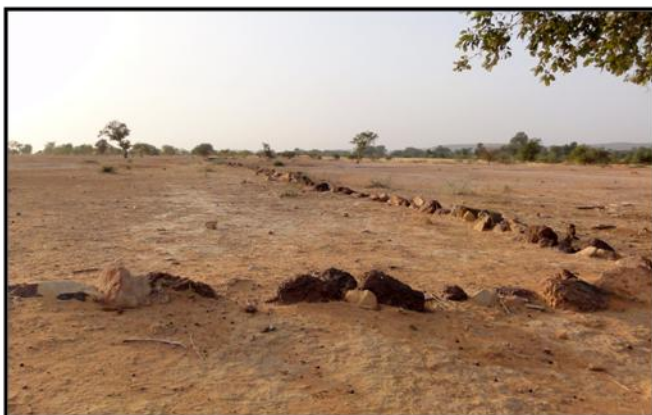
Fig.4.17: Retaining walls designed to capture soil and hinder progression of degraded areas west of Diamnati, Dogon Plateau.
